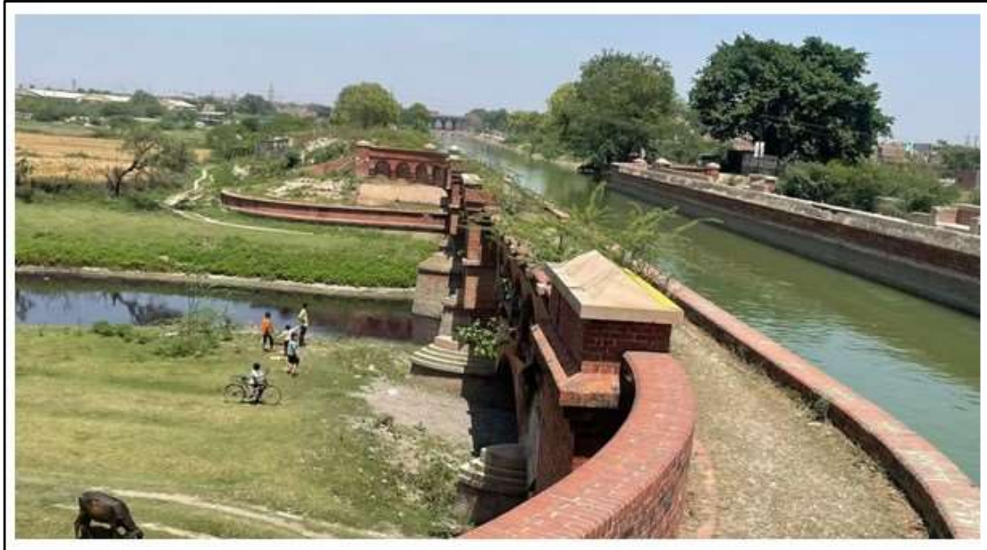
Image-2: Gujaini Aquaduct and Bridge on River Pandu
